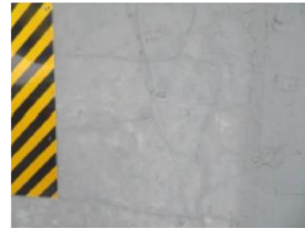
23#墩身小桩号侧网状裂缝
