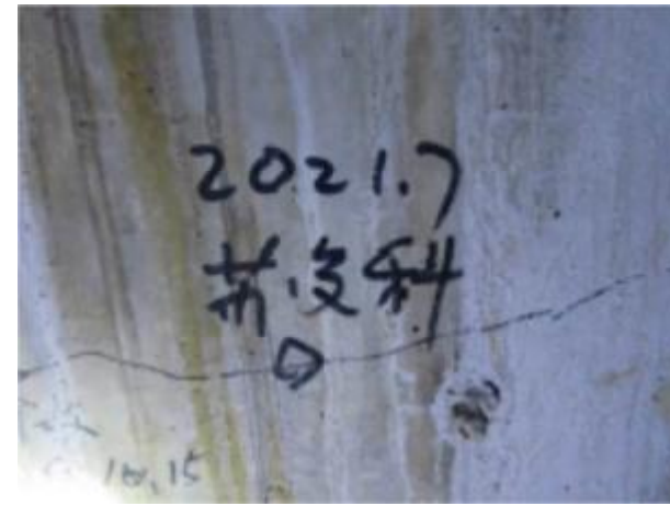
箱室内23#墩顶横隔板竖向裂缝
