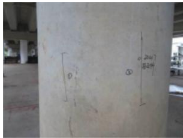
12-2#立柱竖向裂缝
