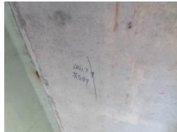
74-4#箱梁底板纵向裂缝
