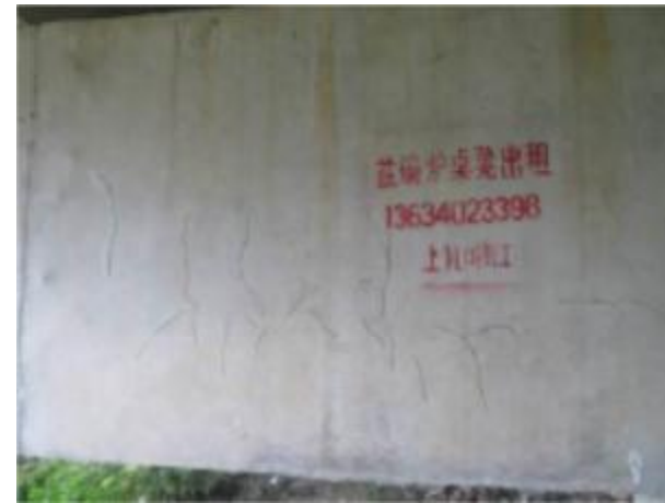
1#盖梁小桩号面网状裂缝
