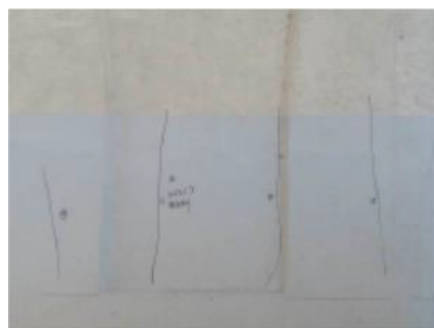
32#墩身小桩号侧竖向裂缝
